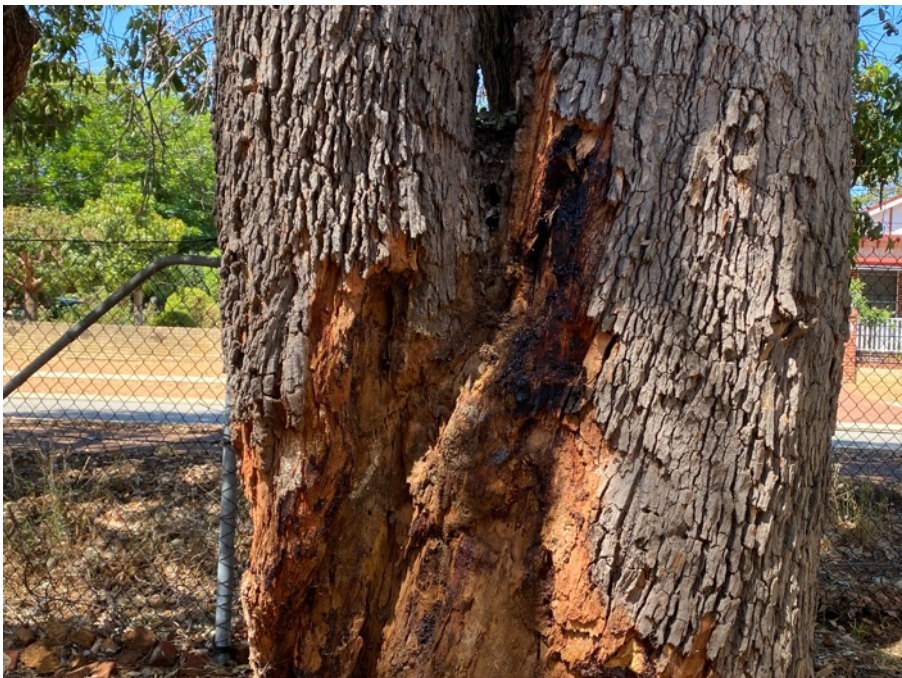
Figure 4. Closer inspection within the large wound revealed wood decay, active termite infestation and additional infection by a resupinate fungus likely to be Macrohyporia sp.; looking towards the east.
