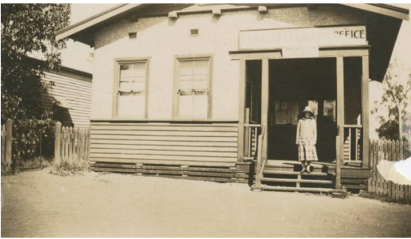
Picture 13 – Post and Telegraph Office, 1925
