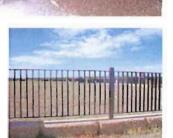
to ensure no potential head entrapment risks for children are created, i.e. no partially bound openings with a lower edge more than 600mm above the ground.
