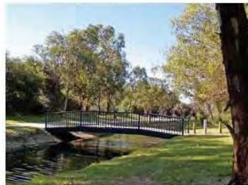
IMAGE 12 Footbridges can be used to provide pedestrian connections
