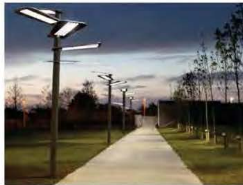
IMAGE 15 Public spaces should be well lit using contemporary lighting solutions
