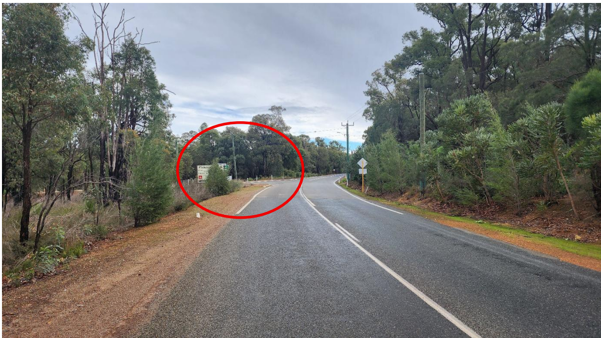
Photo 1: The intersection with the southern Canning Road route is not very visible from the Pickering Road approach.
