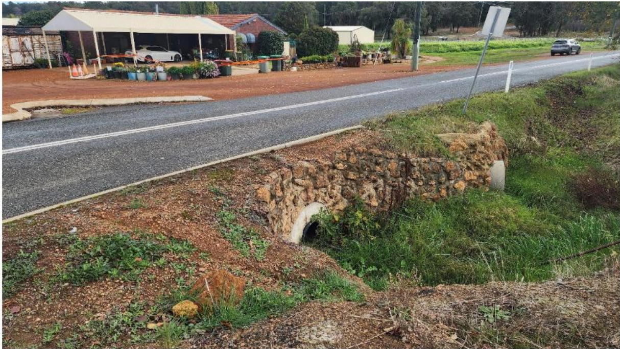
Photo 4: Narrow culvert under Bracken Road, just north of Pickering Brook Road intersection.
