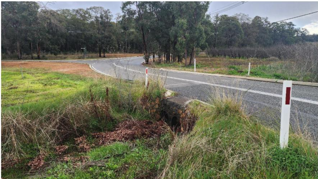
Photo 5: Narrow culvert under Patterson Road, between Bracken Road and Forrest Road intersections.
