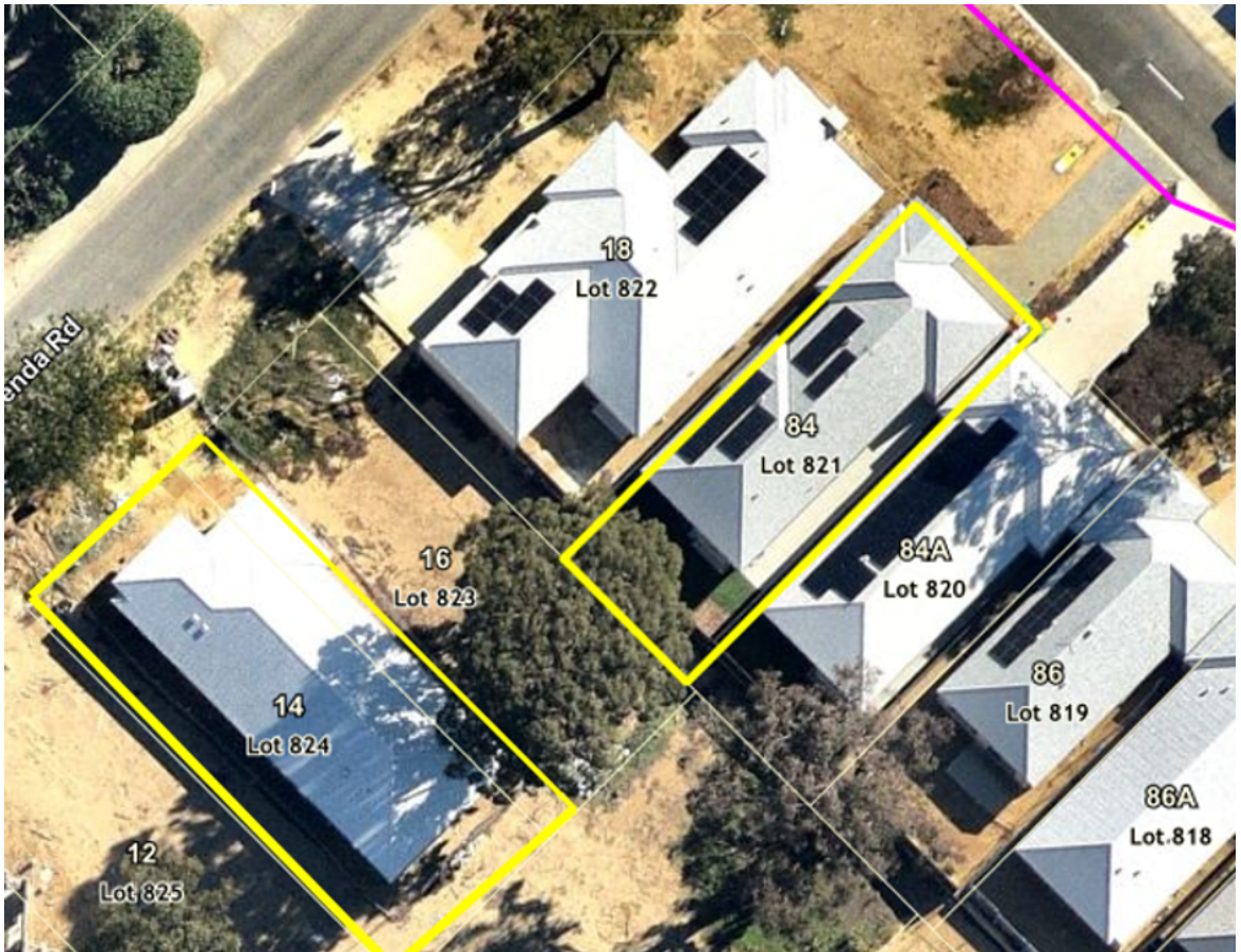
Figure 8: No.14 Brenda and No.84 David street Dwellings constructed while protecting the TPZ of 16 Brenda Road.
