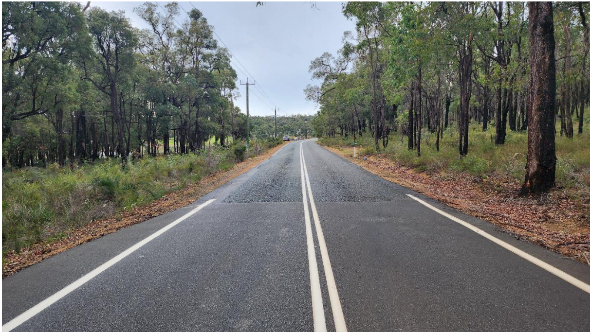
Photo 3: Patterson Road transitions from over 6.0m between edge lines to the south, to a 5.5m seal in the north.
