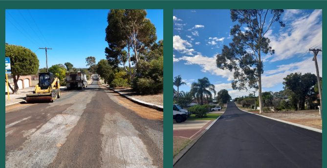
Peter Road profiling and asphalt comp
