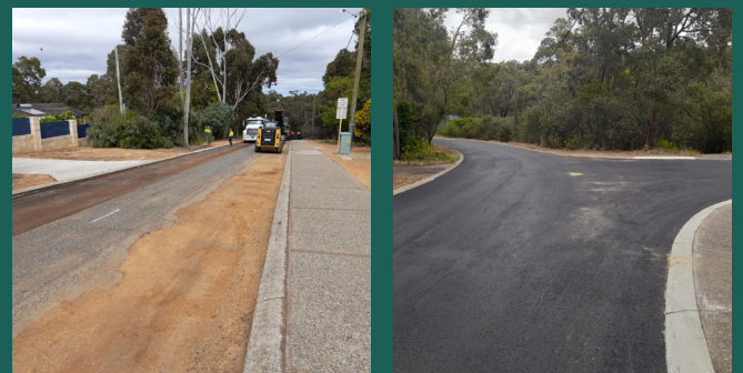
Artthur Road profiling and asphalt comp
