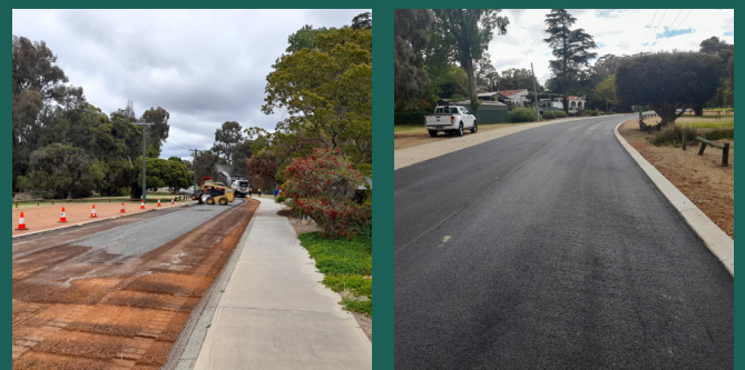
Kaolunga Way profiling and asphalt comp
