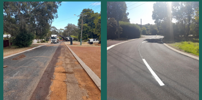
Grace Road profiling and linemarking comp
