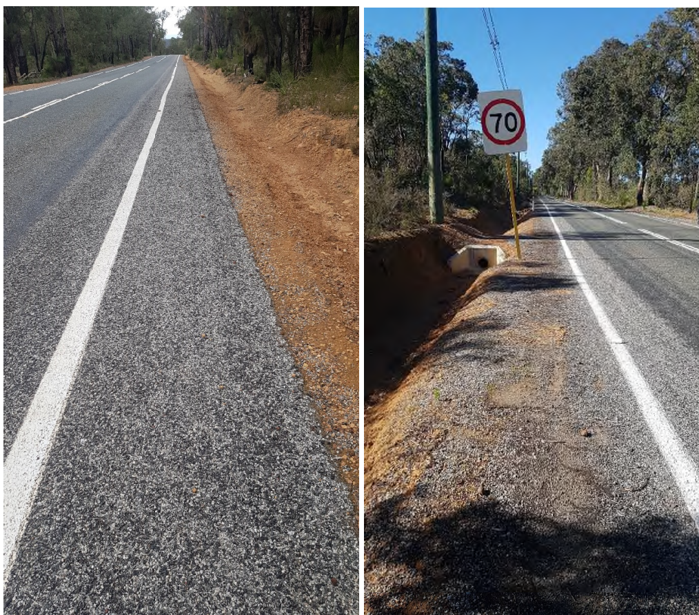
Photos 81 & 81a: Hard shoulders vary in width and rideability. Note temporary reflector tabs on white lining.
