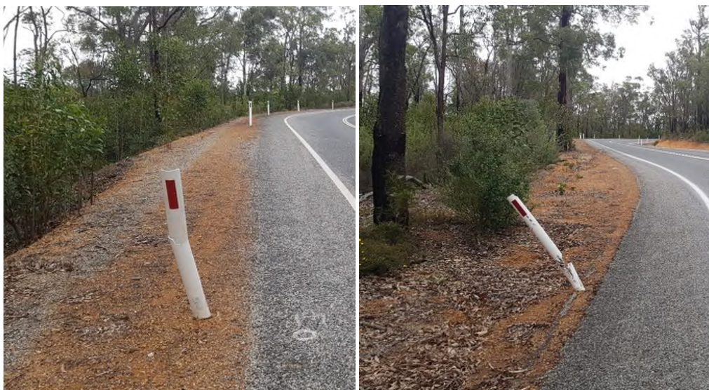
Photos 99 & 99a: Broken guide posts.
