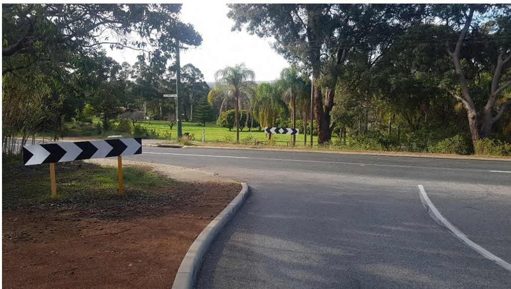
Photo 30: Side road approach has no Give Way signs or lines.
