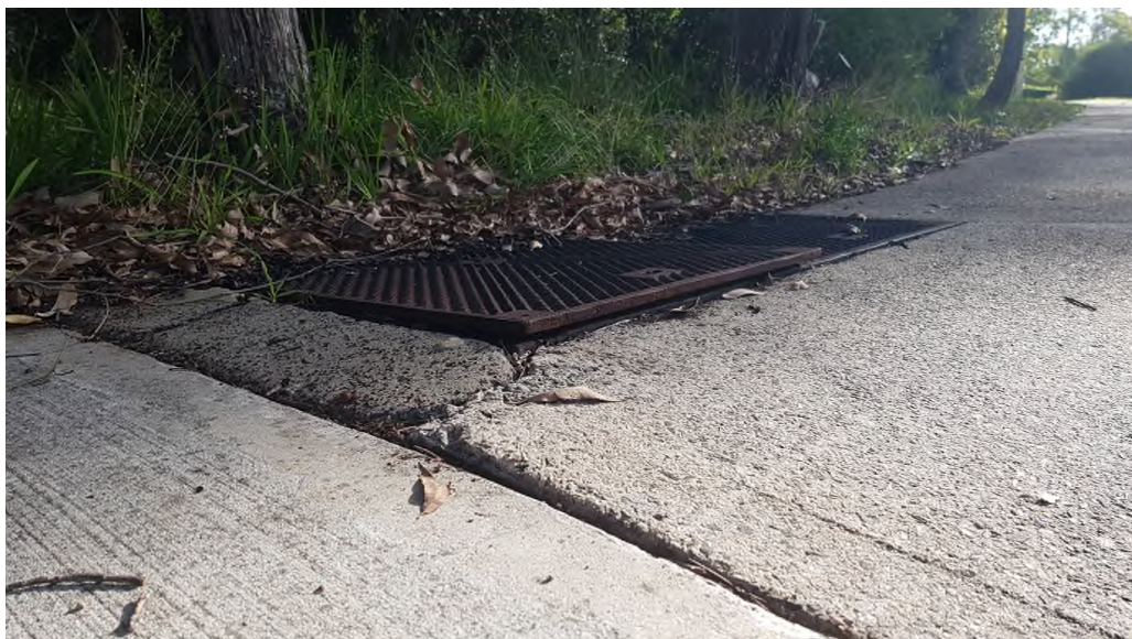
Photo 71: Trip hazard in footpath.
