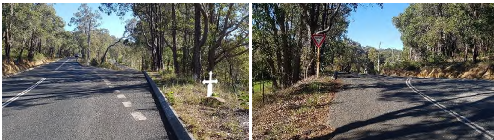
Photos 35 & 35a: Northern of the two Aldersyde Road connections forms an acute Y-intersection.
