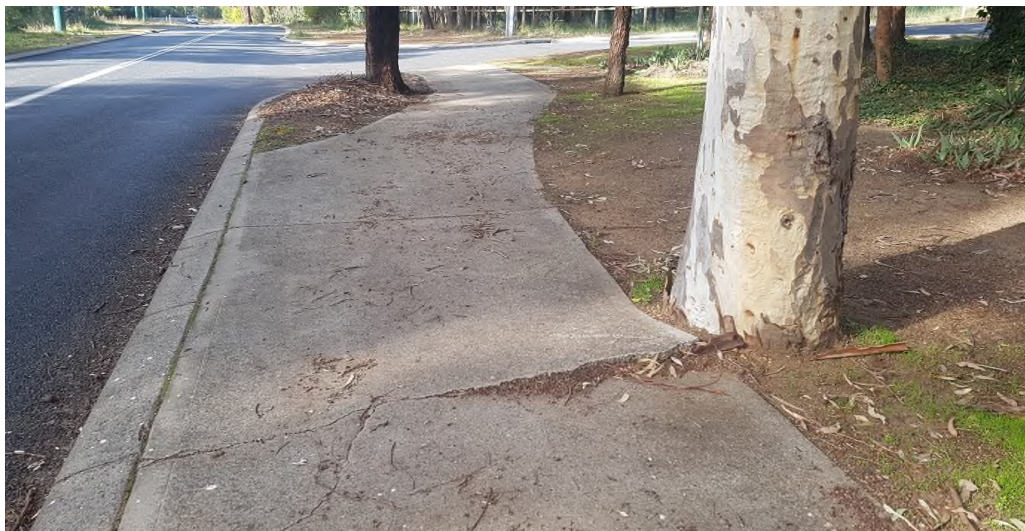
Photo 72: Significant trip hazard due to root damage.
