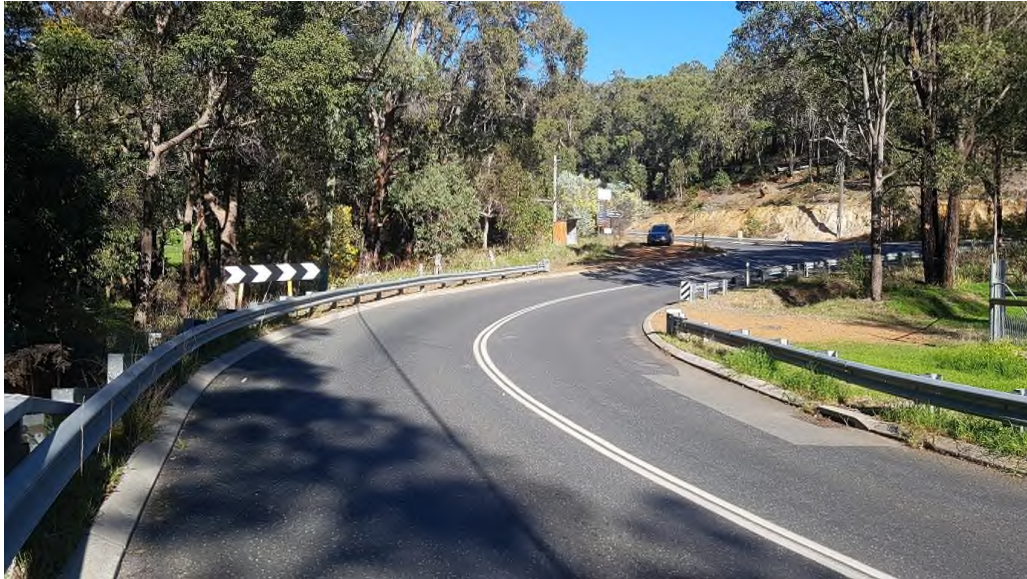
Photo 13: This bend has a radius of approximately 35m.
