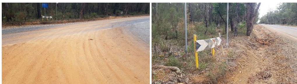
Photos 49 & 49a: Loose material being dragged onto the carriageway and a damaged (incorrect) hazard board.
