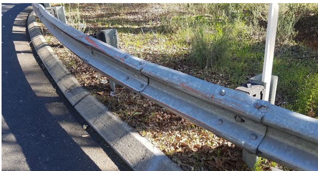
Photo 39: Safety barrier is very close to kerb line and has been struck several times.
