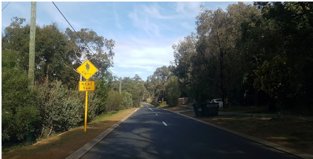
Photo 87: One example of a number of sign faces that are worn and consequently no longer retro-reflective.
