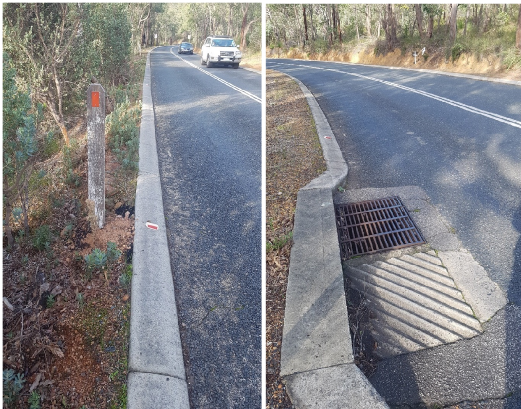
Photo 90: Very old guide post. Note reflectors mounted on kerbs. Photo 91: Non-cycle friendly drainage grid.
