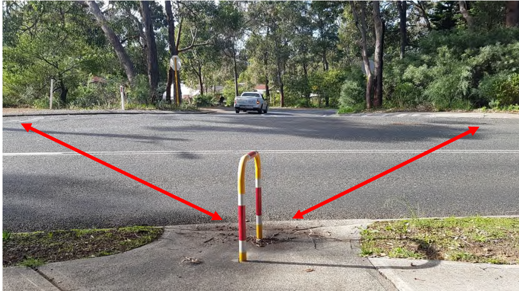
Photo 70: The crossing is badly aligned, with ramps well below current standards, no TGSIs and limited visibility.
