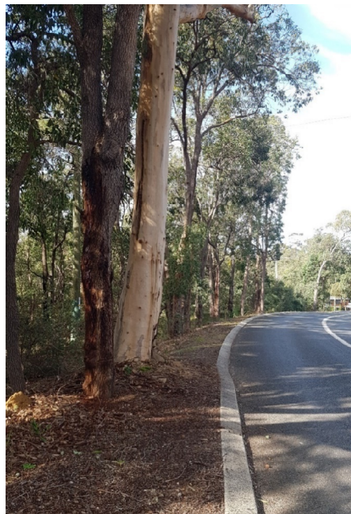
Photos 84 & 84a: Roadside hazards for errant vehicles include non frangible power poles and trees.
