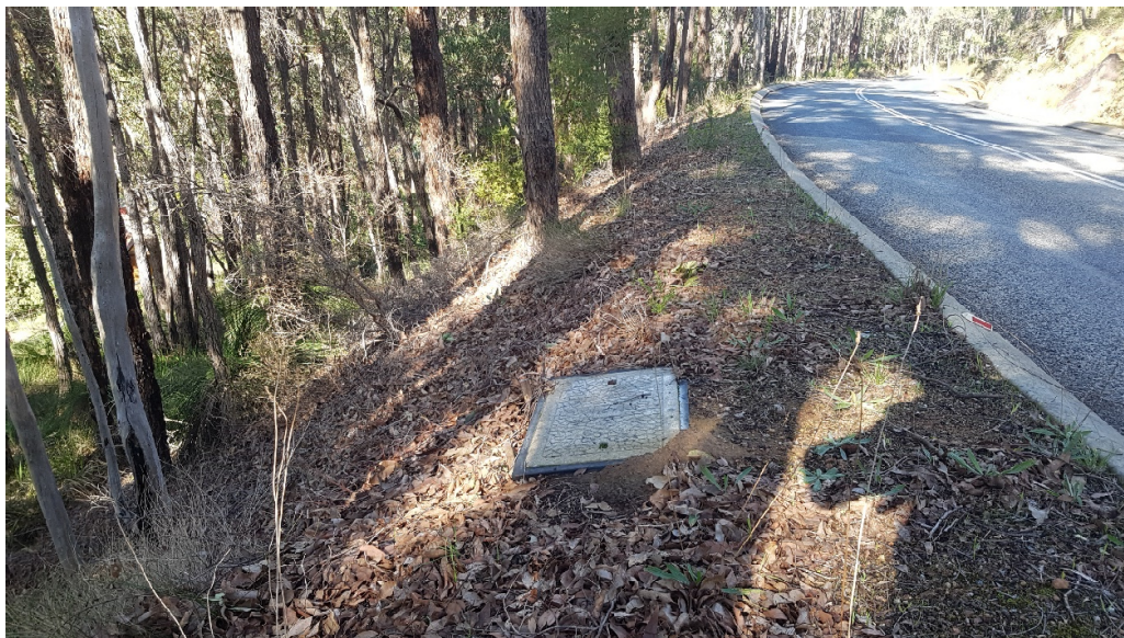
Photo 88: Unrecoverable batter with a significant drop off. Note service lid.
