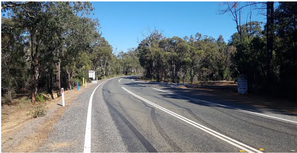
Photo 44: Visibility to the right from the Paulls Valley Road intersection is limited by a horizontal curve.
