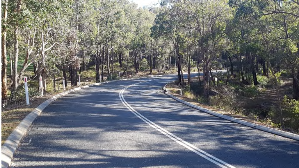
Photo 11: This bend has a radius of around 55m.
