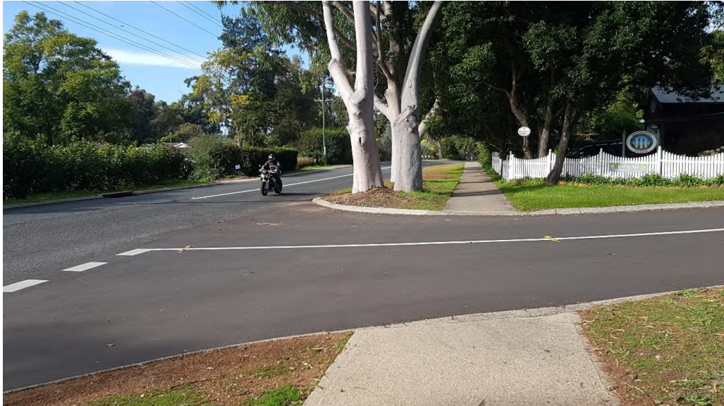
Photo 68: Typical pedestrian crossing, with ramps being well below current design standards.
