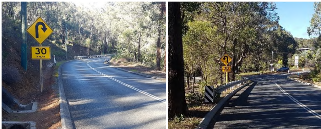
Photos 14 & 14a: Advisory speed signs installed on both approaches.
