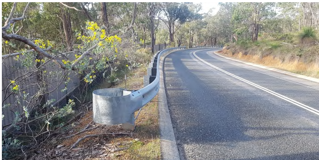
Photo 92: W-beam with a non-crashworthy termination treatment.
