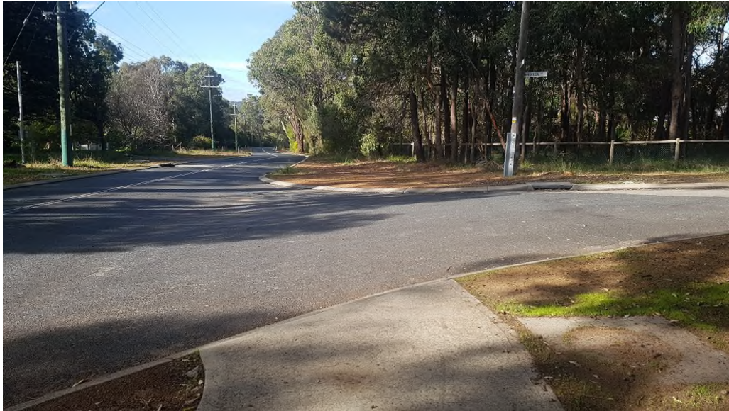
Photo 77: The footpath terminates at this point, with no continuation along either road.
