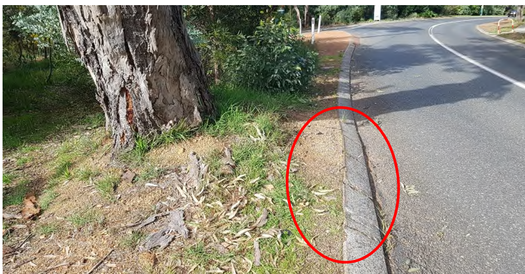
Photo 85: Tree roots are beginning to lift and crack the kerbs.
