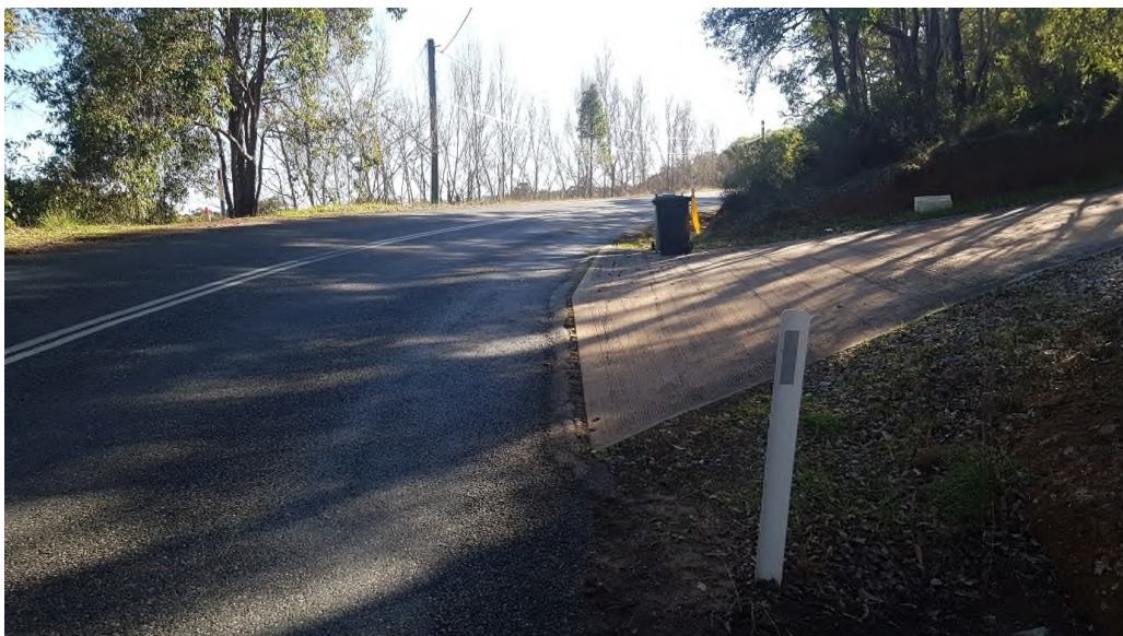
Photo 62: Steep concrete driveway on inside of curve gives limited visibility.
