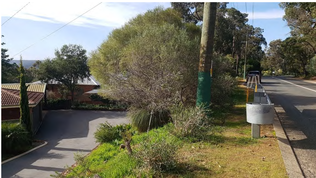
Photo 83: Barrier is too short, does not fully protect the power pole and has non-crashworthy end treatments.
