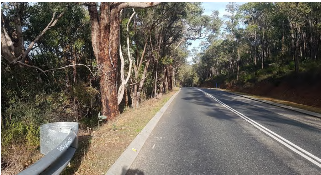
Photo 94: Although the safety barrier ends here, the roadside hazards do not.
