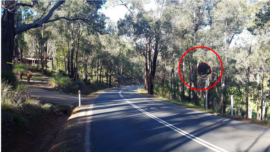
Photo 63: Convex mirror installed to assist with visibility.
