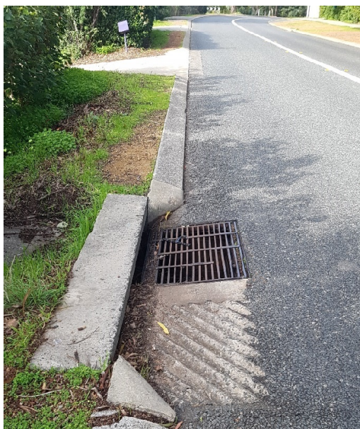
Photo 76: Typical 'Cycle-unfriendly' drainage facility.
