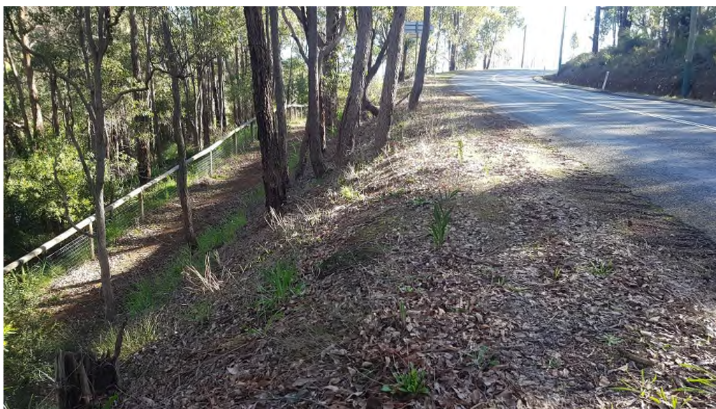
Photo 89: Another typical drop off along this section.
