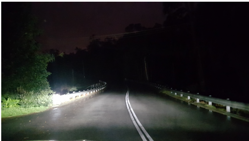
Photo 105: The alignment through the bridge is not well delineated at night.
