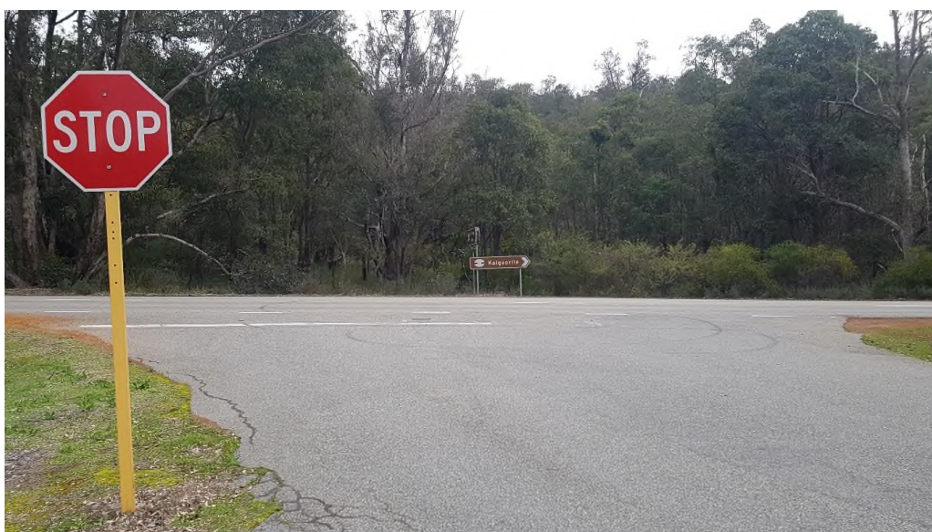
Photo 60: The access is not kerbed, but does have a Stop sign and line.
