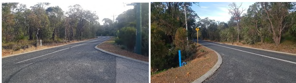
Photos 34 & 34a: Visibility is limited in both directions by bends in the through road.
