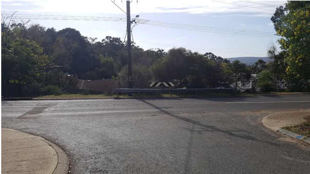
Photo 22: Hazard board, but no Give Way lines or signs. Note unsuitable safety fence.
