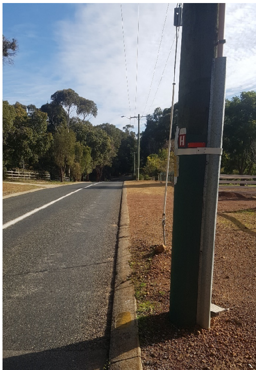
Photos 84 & 84a: Roadside hazards for errant vehicles include non frangible power poles and trees.
