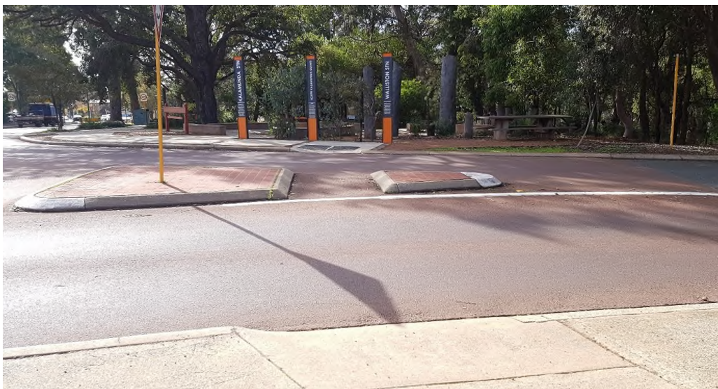
Photo 67: Tactile Ground Surface Indicators (TGSIs) are poorly aligned or missing.
