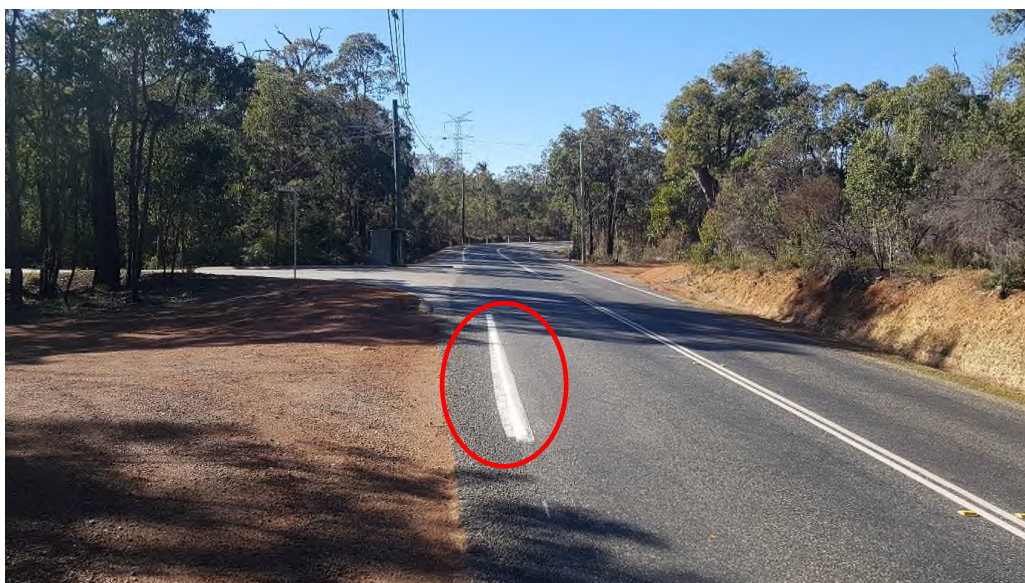
Photo 40: Fern Road intersection, with non-standard edge line marking.
