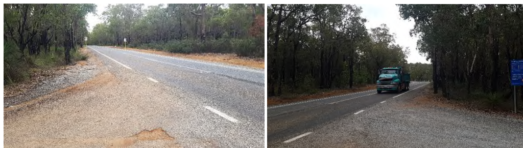
Photos 53 & 53a: The side road radii are not kerbed.
