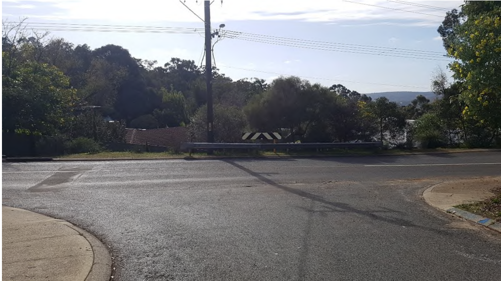
Photo 82: Schmitt Road: No Give way signs or lines. Note unsuitable use of not-to-standard W-beam.
