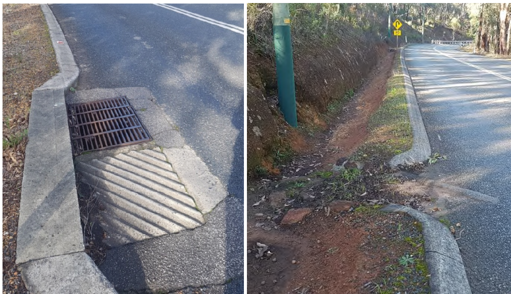
Photos 79 & 79a: These drainage designs present a hazard to cyclists.
