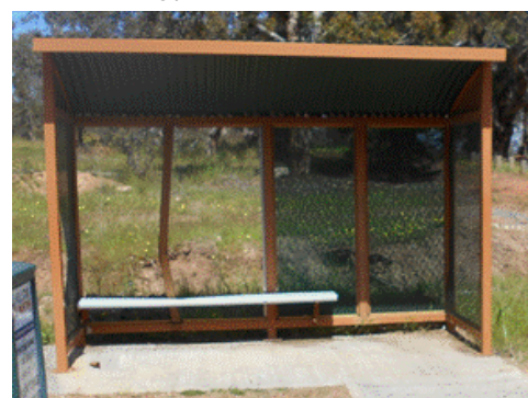
Steel bus shelter (Miricale) with vandalised panels
