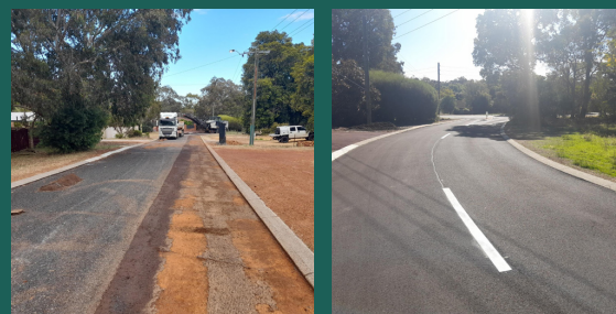
Grace Road profiling and linemarking comp
