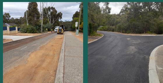
Arthur Road profiling and asphalt comp
