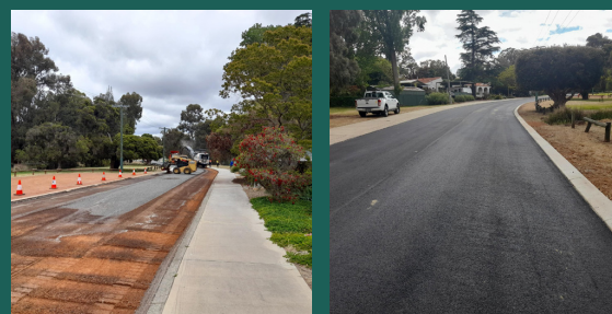
Kaolunga Way profiling and asphalt comp
