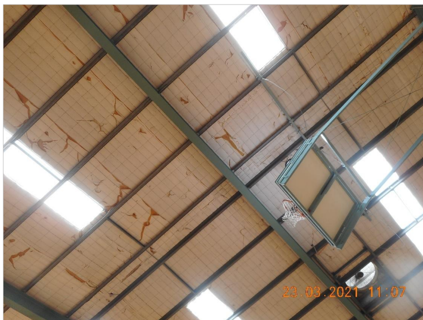
Replacement of roof sheeting and lining
