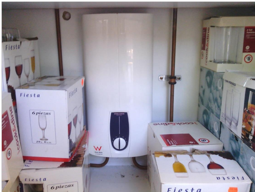
Replacement of water heating units
