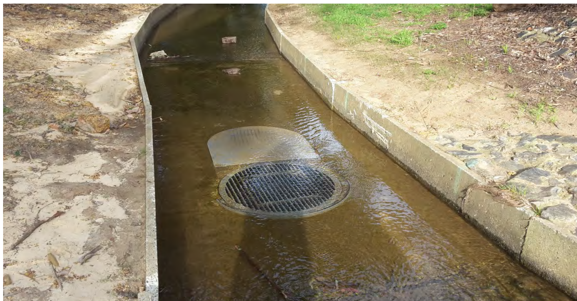
Woodlupine Main Drain stormwater extraction point
