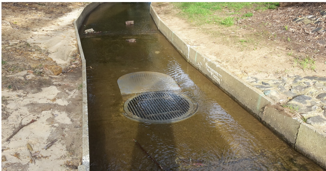
Woodlupine Main Drain stormwater extraction point
