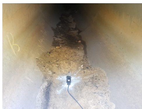
Doppler Sensor installed at Crumpet Creek
