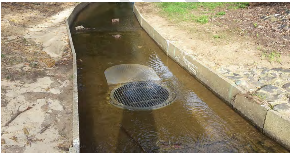
Woodlupine Main Drain stormwater extraction point
