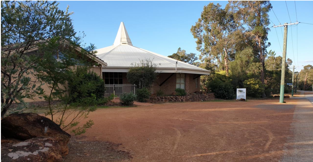
Figure 3: Existing LBC from Brady Road
