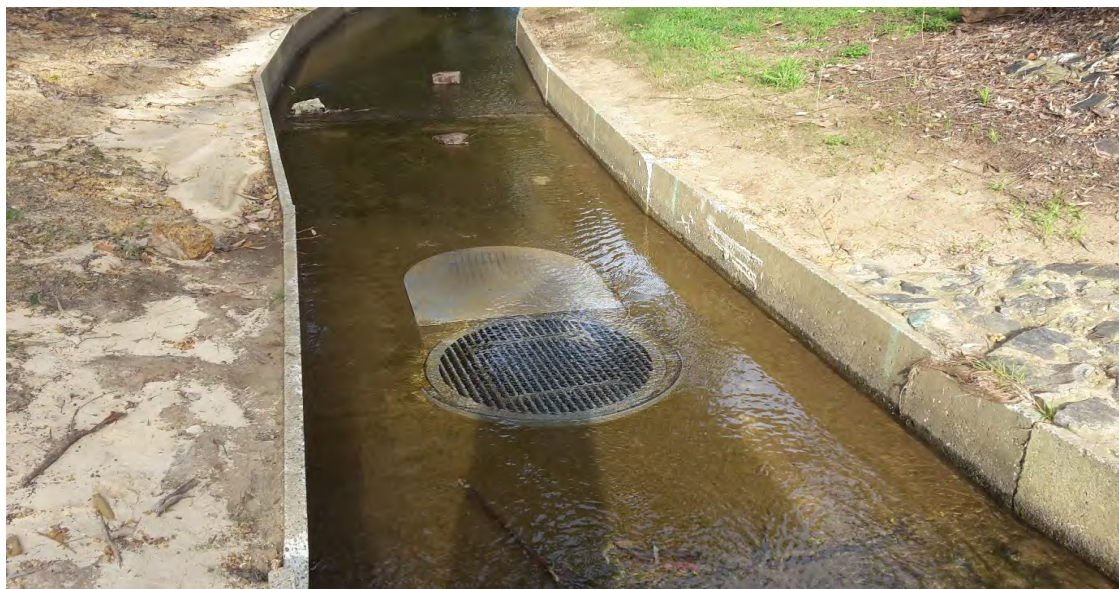
Woodlupine Main Drain stormwater extraction point
