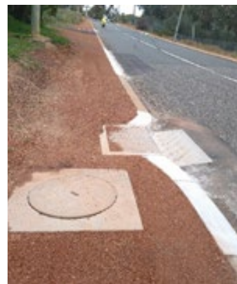
Holmes Road drainage upgrade
