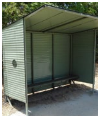
Bus Shelter - after
