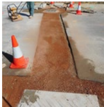
Berberis Way drainage upgrade
