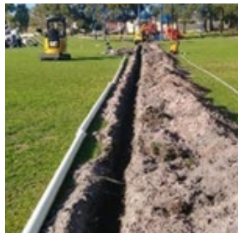
Ollie Worrell Reserve Reticulation Replacement - Mainline installation in progress
