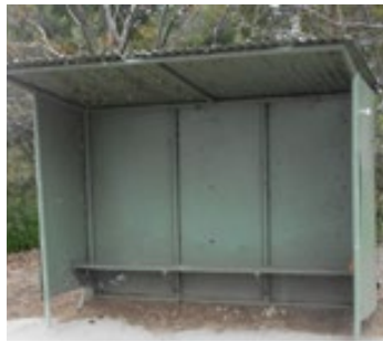
Bus Shelter - before
