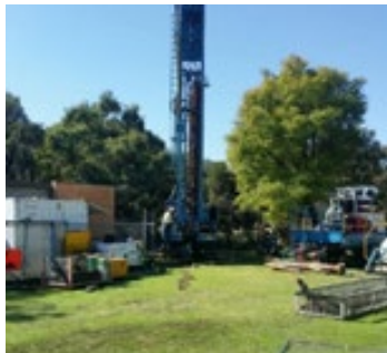
Dedicated injection bore being drilled at the MAR
