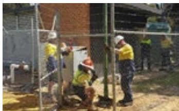
Carbon filters and injection pipework being installed at the MAR
