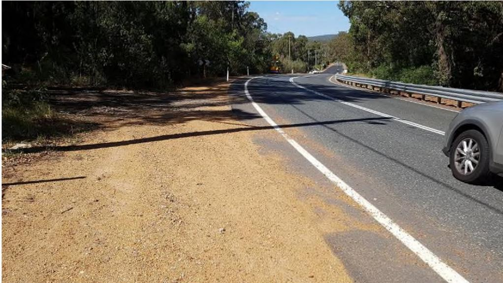
**Photo 34: Loose material on hard shoulder and road surface.**
