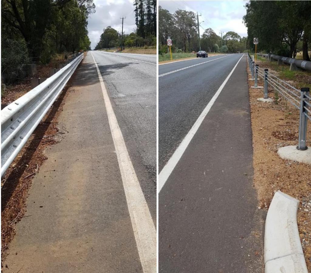
**Photos 22 & 22a: Sealed shoulders are of sufficient width for cyclists to use, but are not to cycle lane standard.**
