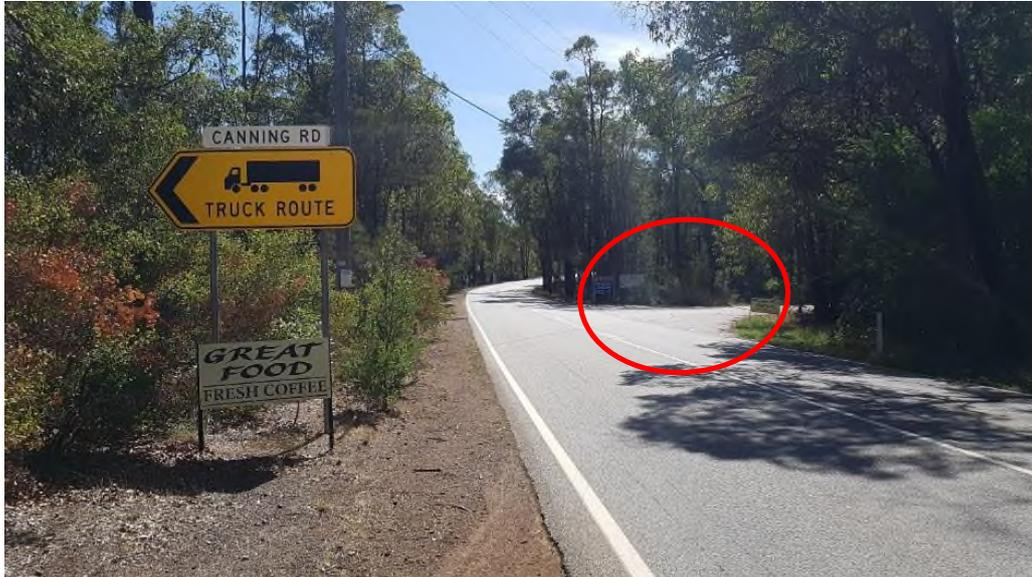
Photo 51: This intersection has no warning signs and very poor visibility.
