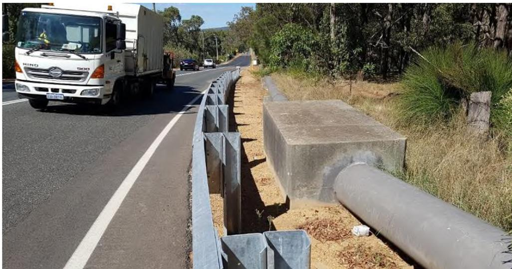
**Photo 33:** If struck by a vehicle, this safety fence may deflect further than the concrete block.
