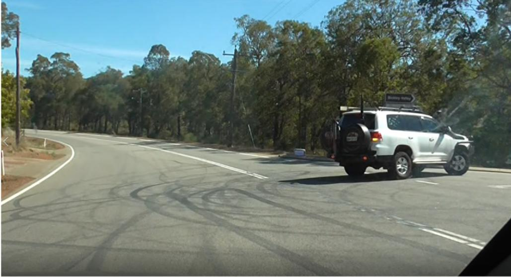
**Photo 12: Sight distance is limited for right turning vehicles.**
