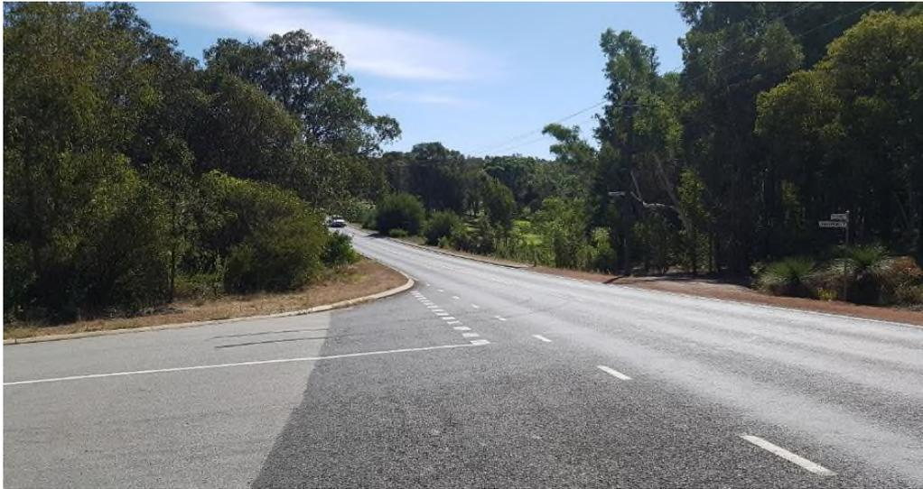
**Photo 36:** Visibility to the north is limited by both geometry and roadside vegetation.
