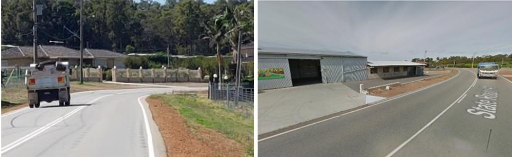
**Photos 44 & 44a:** There are a number of property accesses around blind bends. Leotta's access provides one example.
