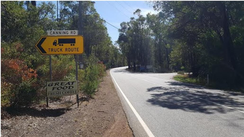
**Photo 16:** Intersection with an unnamed link road, looking north. Note lack of warning signs.
