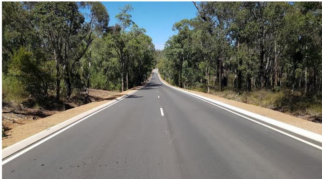
**Photo 28: No hard shoulder between edge lines and kerbs.**
