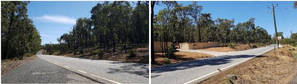
**Photos 40 & 40a:** Northern service road intersection joins Canning Road at an acute angle of around 20°.
