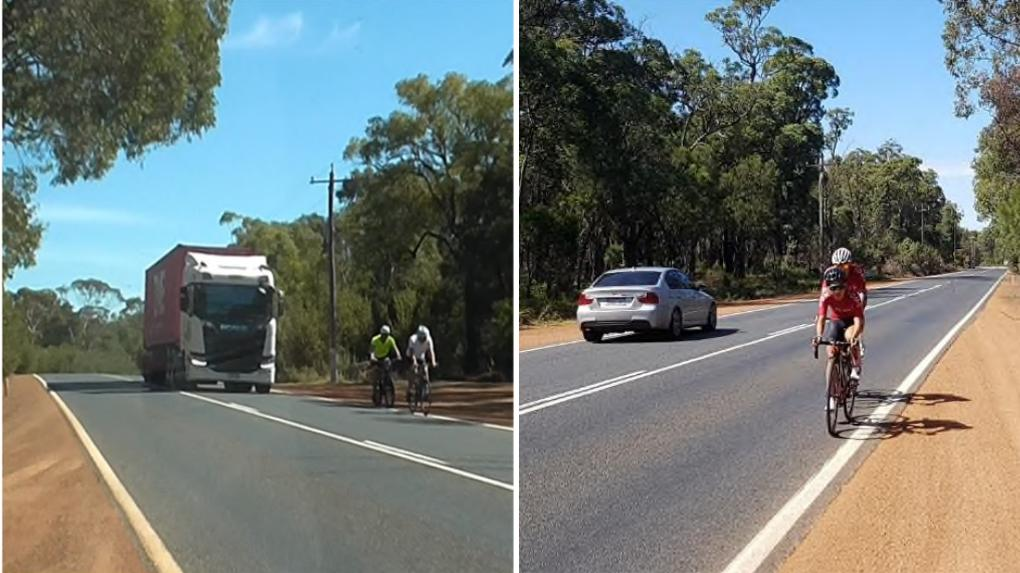
**Photo 25 & 25a:** The lack of sealed shoulders force cyclists to share the road space with other vehicles.
