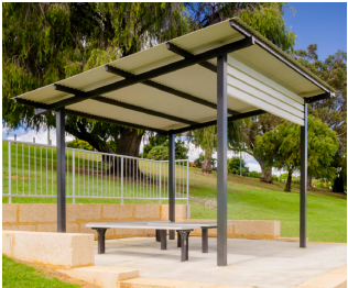
Shade shelter with seaing and drinking fountain
