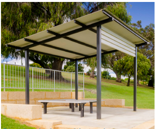
Shade shelter with seaing and drinking fountain
