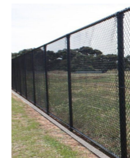
Fence with flush 150mm concrete strip beneath
