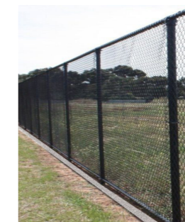
Fence, with flush 150mm concrete strip beneath
