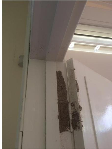
Figure 128 Sunroom, termite damage
