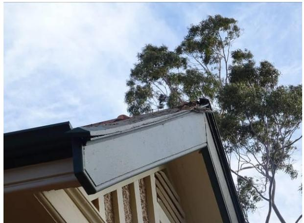
Figure 26 Damaged timberwork to gable end
