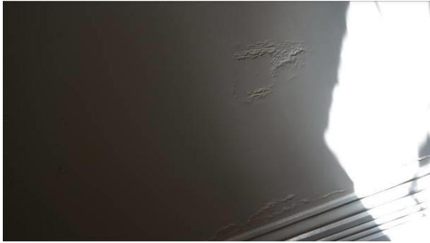
Figure 64 Main entry, evidence of damp
