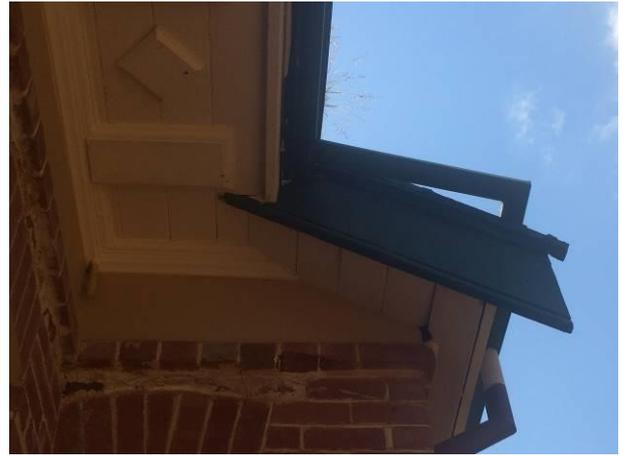
Figure 14 Exposed downpipe in gutter
