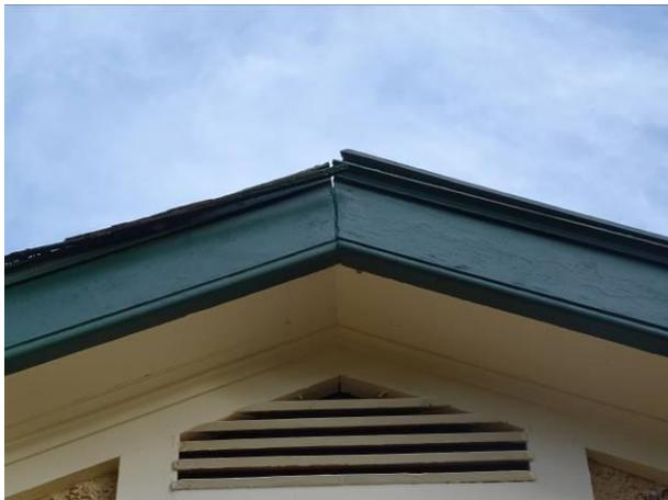
Figure 25 Damaged timberwork
