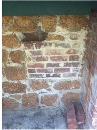
Figure 35 brick patch to wall behind condenser units
