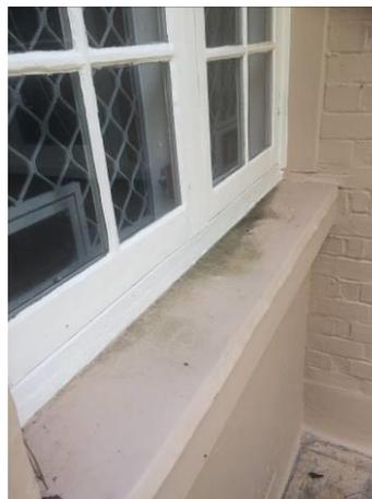
Figure 43 pressed metal capping to sill
