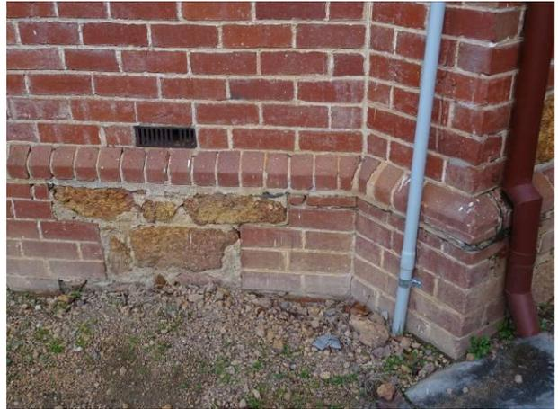
Figure 24 Fretted & damaged brickwork
