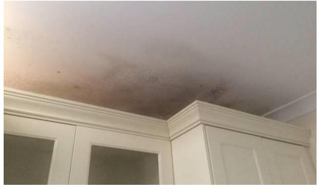
Figure 102 Water staining to ceiling of kitchen
