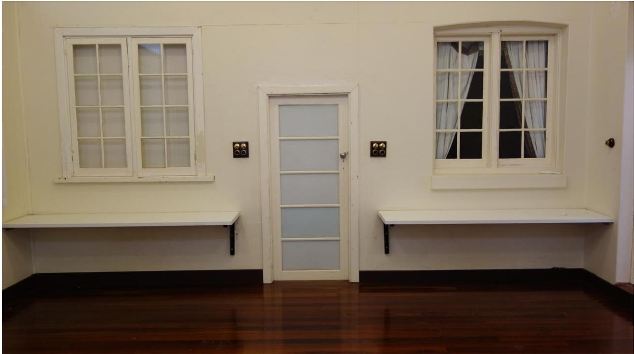
Figure 131 Existing opening proposed to be modified for new floor level and universal access.
