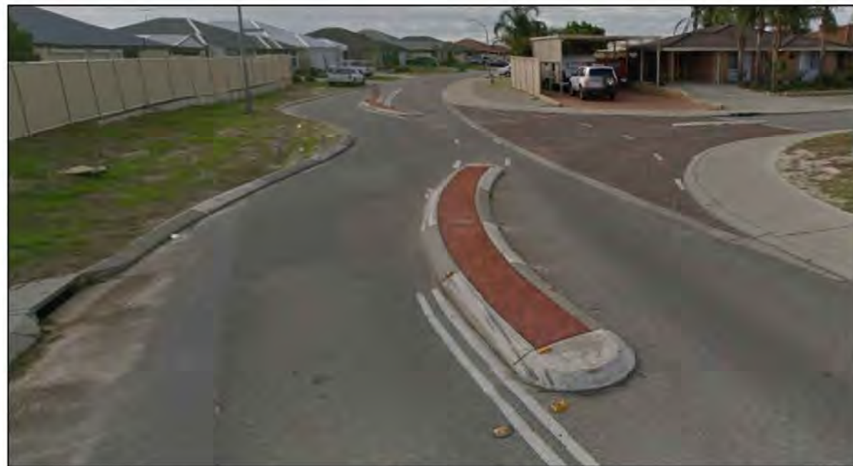
PHOTOGRAPH TYPICAL INSTALLATION OF A MODIFIED 'T' INTERSECTION
