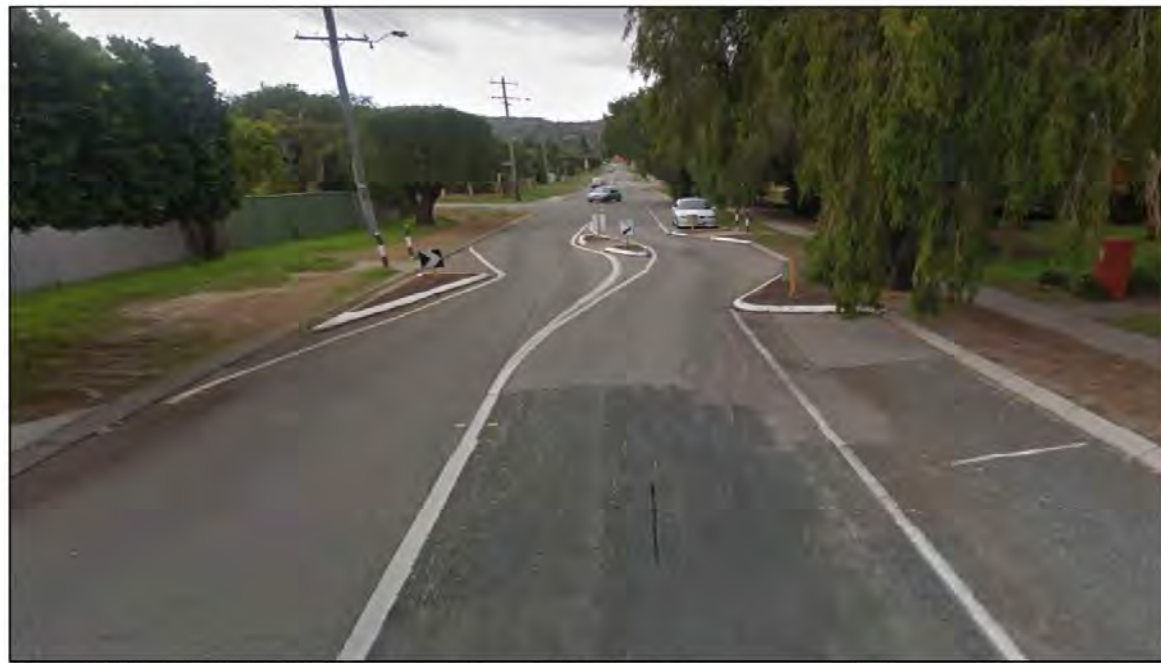
PHOTOGRAPH TYPICAL INSTALLATION OF A TWO LANE SLOW POINTS
