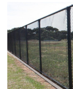
Fence with flush 150mm concrete strip beneath
